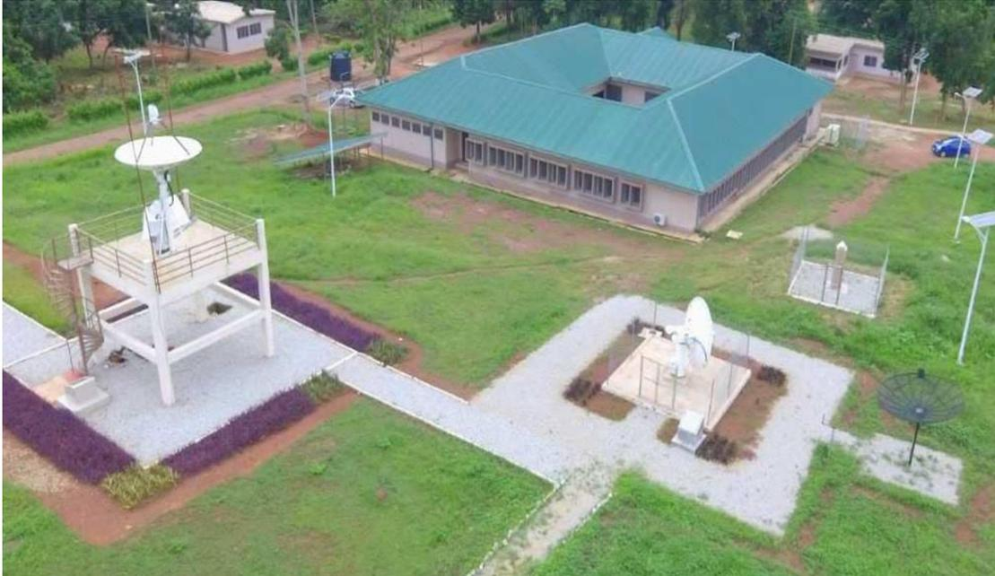
Figure 81: GNSS referencing station mounted at the compound of the University Energy and Natural Resources
