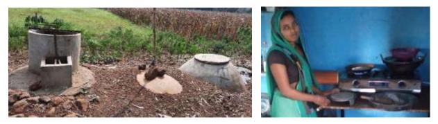
Millions of household biogas plant converts animal dung and agro-waste into methane gas and good quality manure through anaerobic digestion process. The Methane gas produced by the biogas plants is used for cooking as a clean fuel in rural areas while the degassed manure is used for organic
