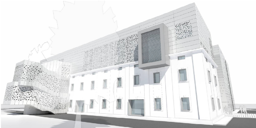
Picture 4. Three-dimensional view of the old building with the implemented dual-layer, segmented façade
