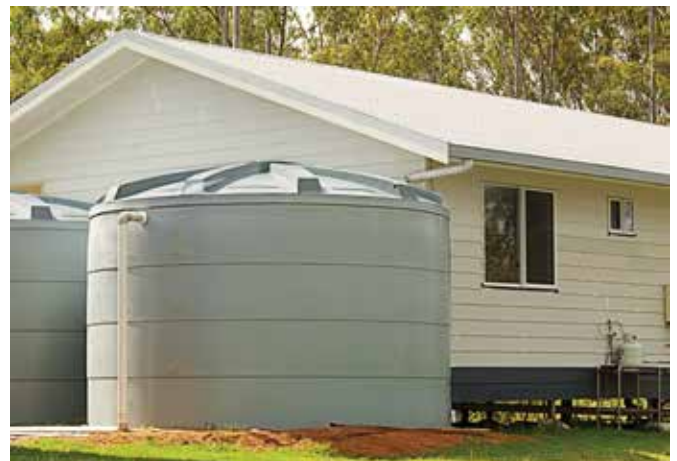
Image 3: Rainwater conservation tanks on new house in Australia
