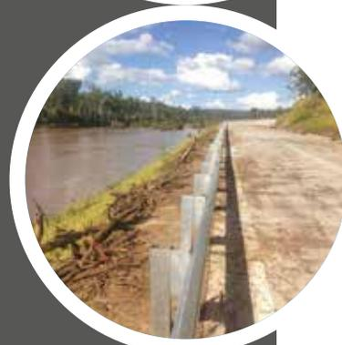
The Betterment project has rebuilt and increased the resilience of the two-kilometre section of road adjacent to the Burnett River that was washed out by relocating it uphill by up to 11 metres and installing concrete lined channels, culverts and scour protection.
